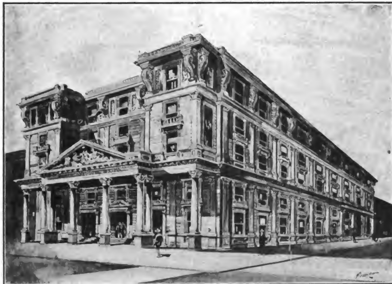
NATIONAL BANK OF CUBA, HAVANA. New Building Now Under Construction.
